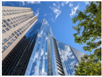
The Winthrop Center and 75-101 Federal St. towers are seen on Oct. 1, 2025. Photo by James Sanna | Banker & Tradesman Staff
