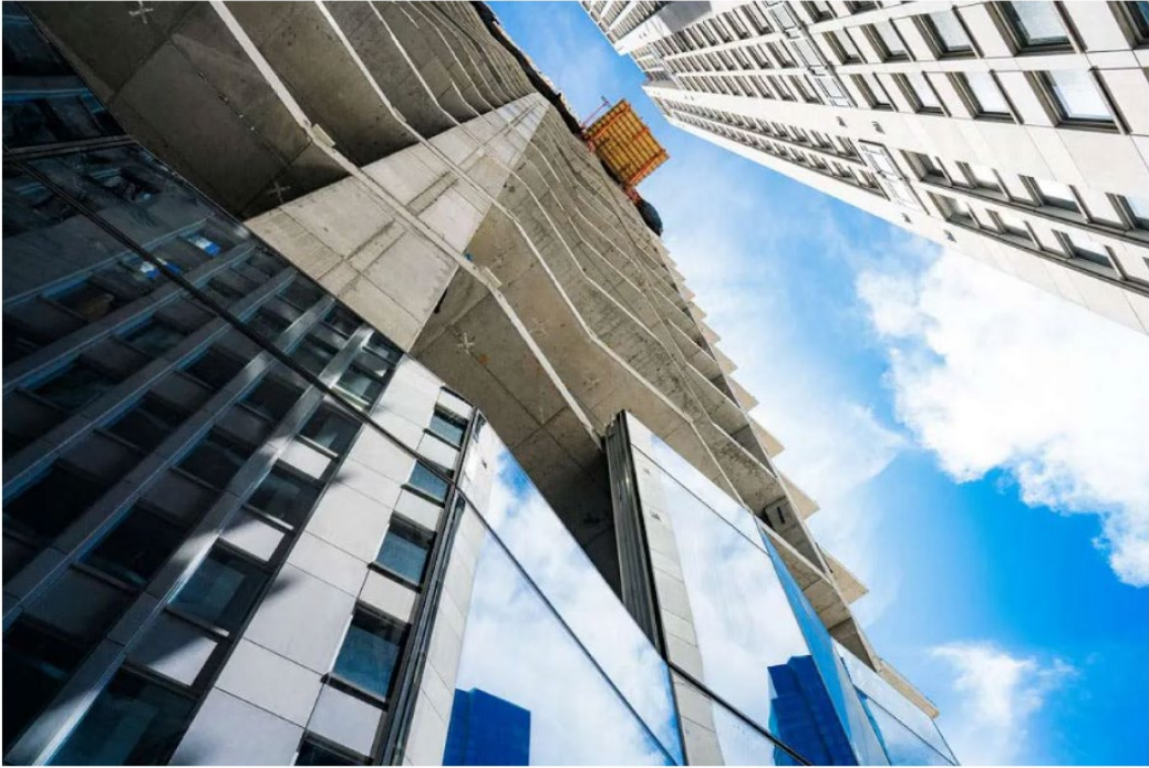
— Windows in Boston's new Winthrop Center help it use 65% less energy and carbon with triple-glazed, high R-value insulated glass. (Image: Millennium Partners)
