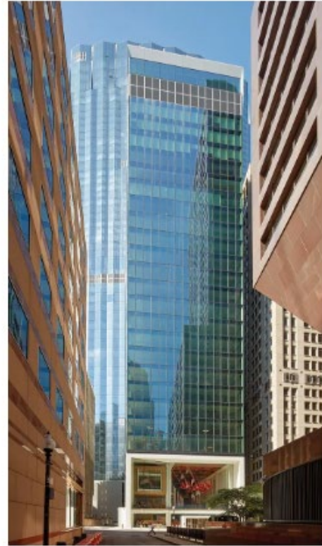
On the tower's west face, the office levels are expressed with a flat, taut skin. Photo © Bruce T. Martin
