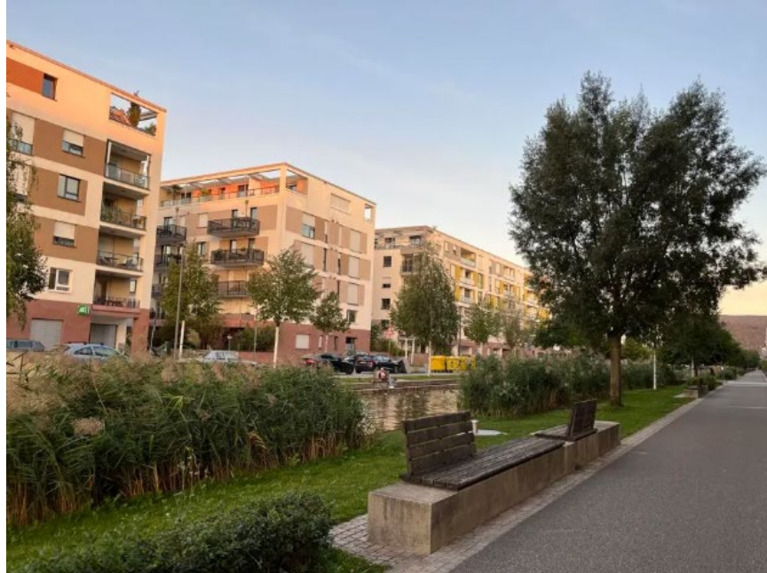
A completed canal section in Bahnstadt
