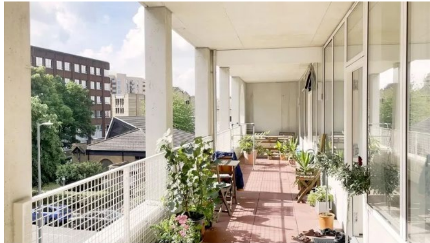
A covered shared balcony that provides shading to the windows
