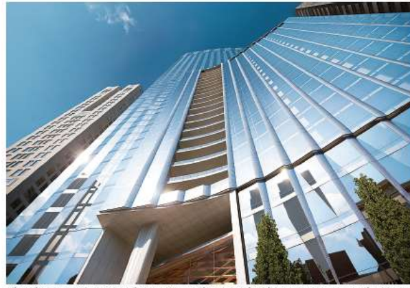
Millennium Partners' 52-story Winthrop Center office and residential tower under construction at 115 Federal St. in Boston is slated to become the world's largest Passive House office building.
