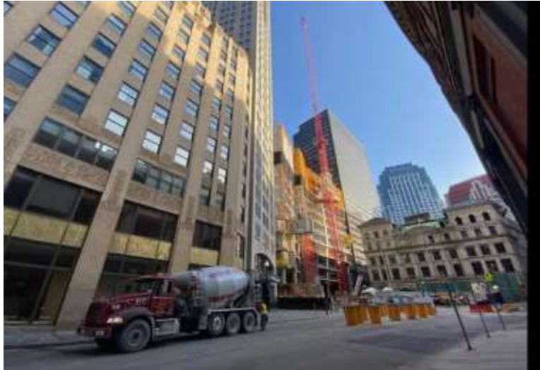
The Winthrop Center rising last week between neighboring buildings.
